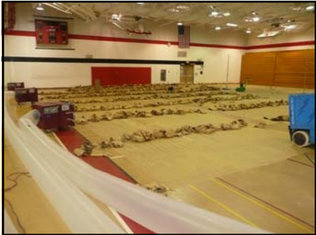
Mercury-Containing Gym Floor Removal
